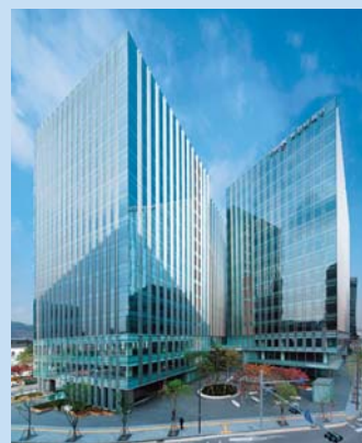
The-K Twin Towers B-13F
