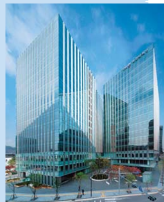
The-K Twin Towers B-13F
